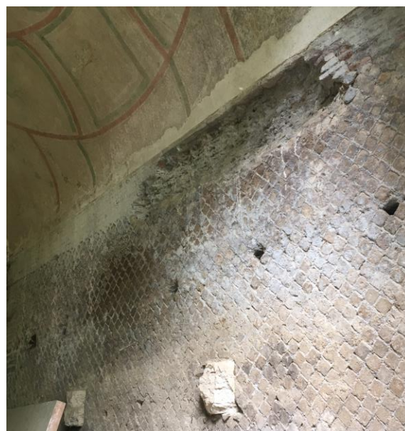
Fig. 17: Hadrian's Villa, western substructure of the Serapeum-Canopus, so-called Tabernae . The interior of the room originally separated by a wooden floor, supported by still existing travertine corbels. Image credits: A. Ottati
