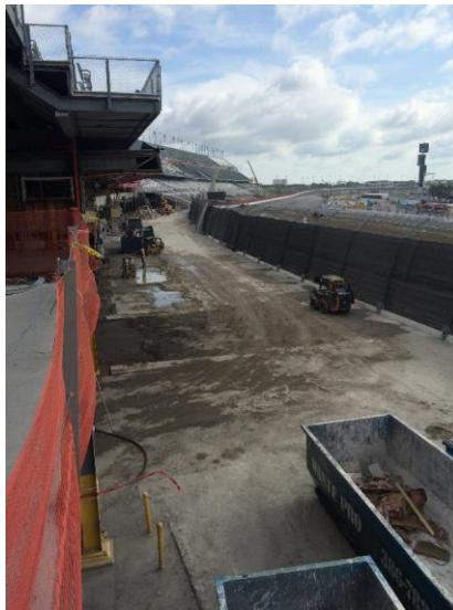
Figure 2: Daytona Speedway - showing partial demolition of the 'frontstretch' seating.
