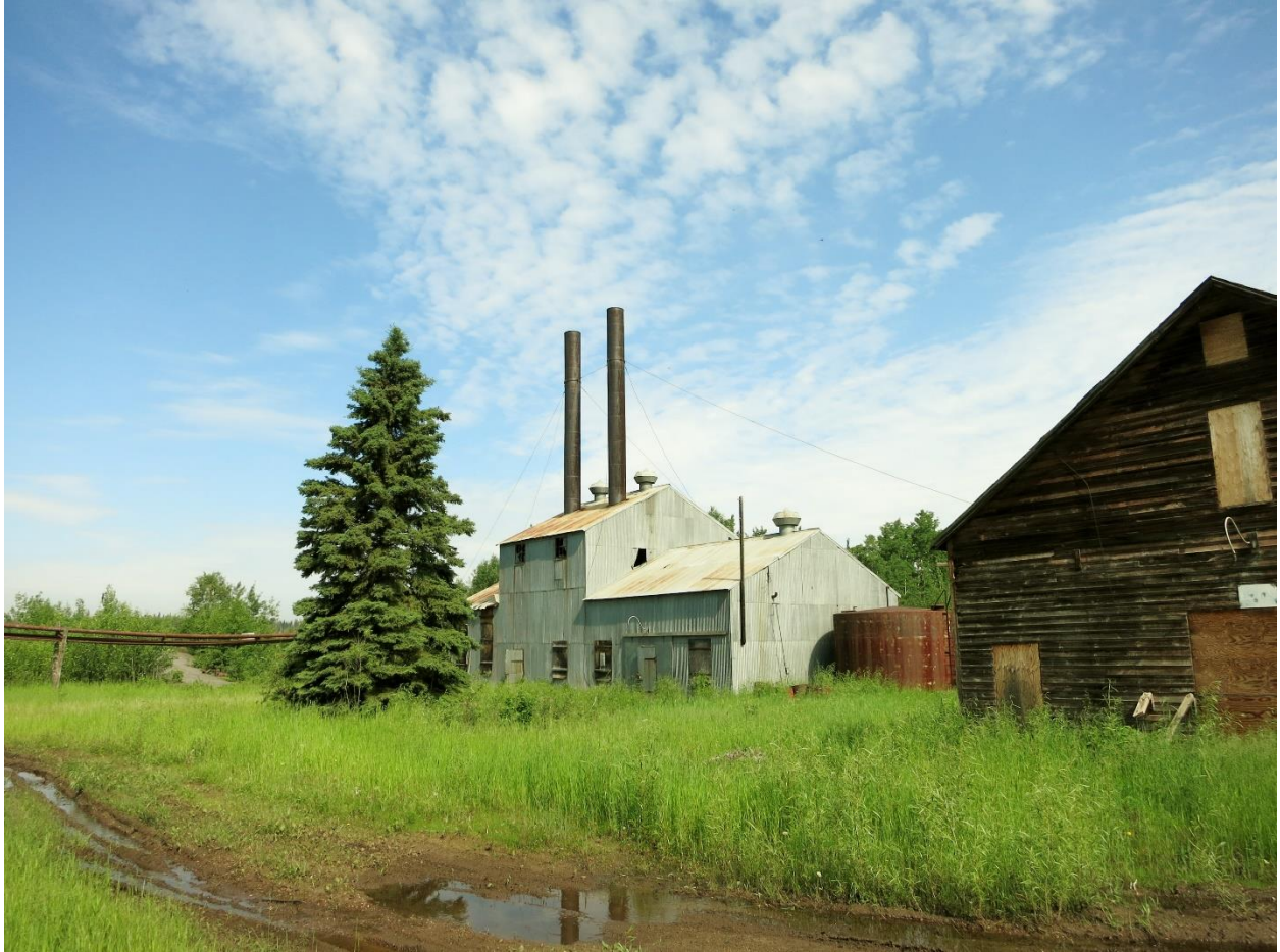
Fig. A.2 The power plant within the processing area at the Bitumount Provincial Historic site, Alberta, Canada (June 2014).
