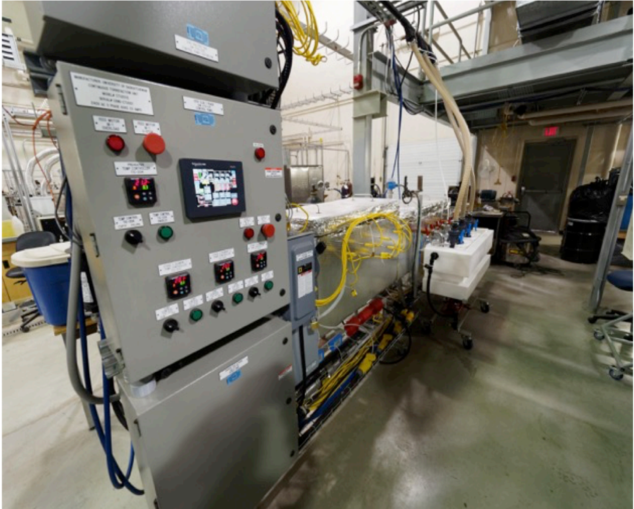
Figure 3.12: Photograph of CTU pilot plant
