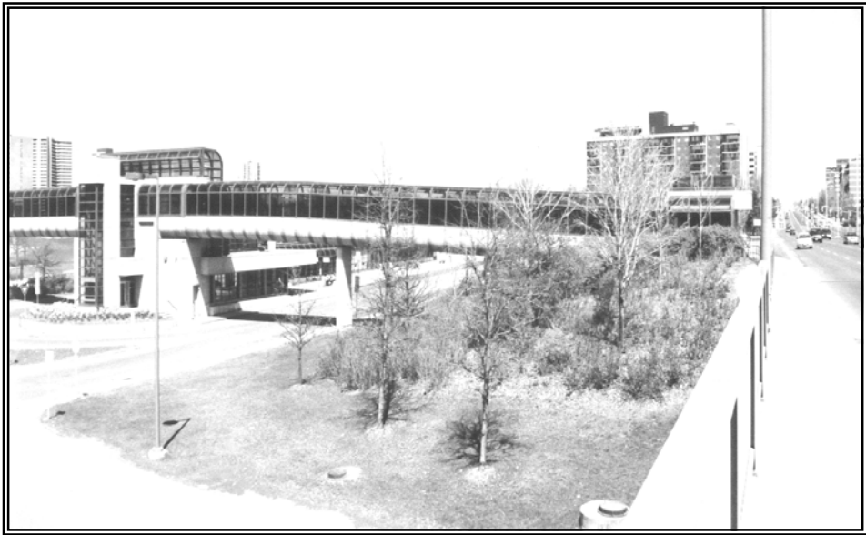
Figure 8.27 Pedestrian Bridge, Lincoln Fields Transitway Station Photo: C. Fullerton
