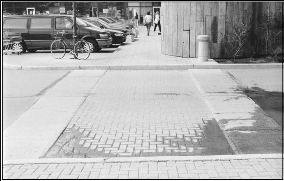
Figure 7.13 Pedestrian Crossing, Orleans Town Centre Photo: C. Fullerton
