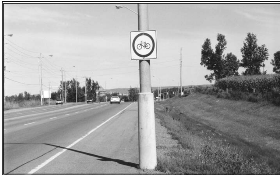
Figure 4.4 Bicycle Lane on Major Arterial Roadway, Ottawa Photo: C. Fullerton
