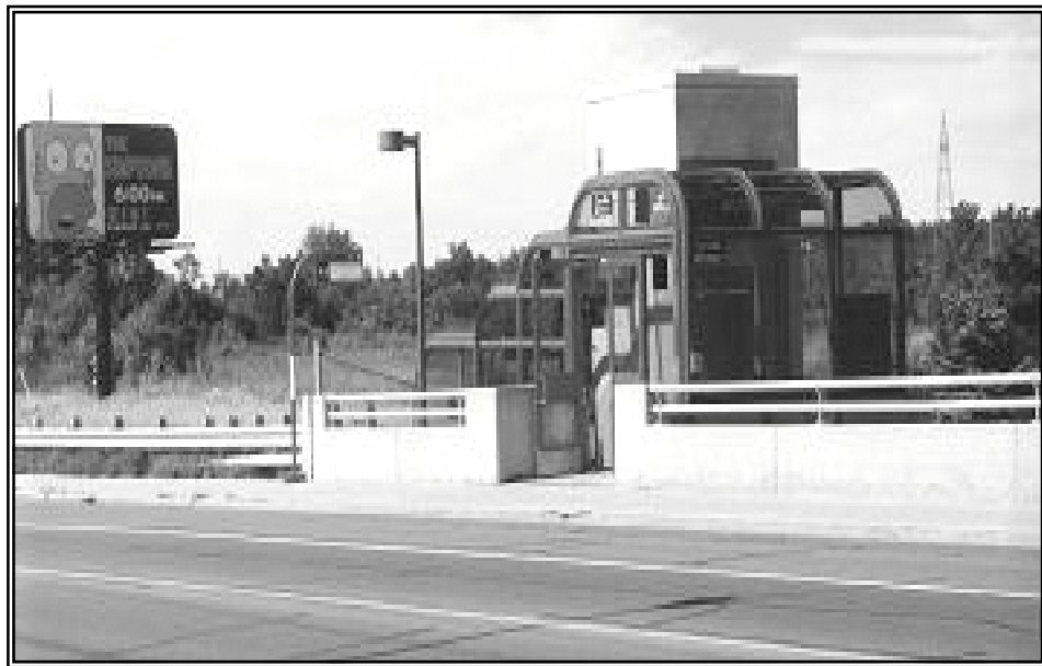
Figures 4.6 and 4.7 Poorly Visible Transit Station, Ottawa Photo: C. Fullerton
