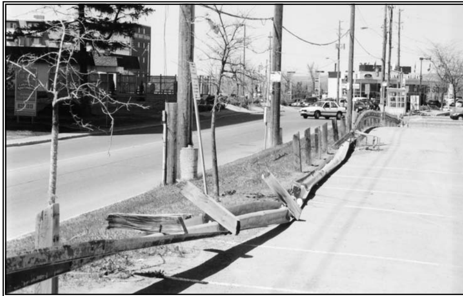
Figure 8.22 Unattractive Waiting Environment, Croydon Avenue adjacent to Lincoln Fields Shopping Centre Photo: C. Fullerton
