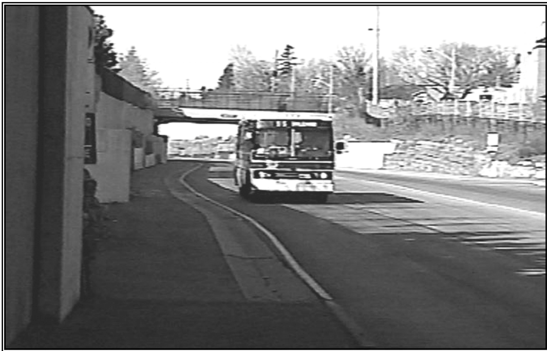
Figure 6.16 Bus Travelling on Ottawa Transitway Source: Williams 2003
