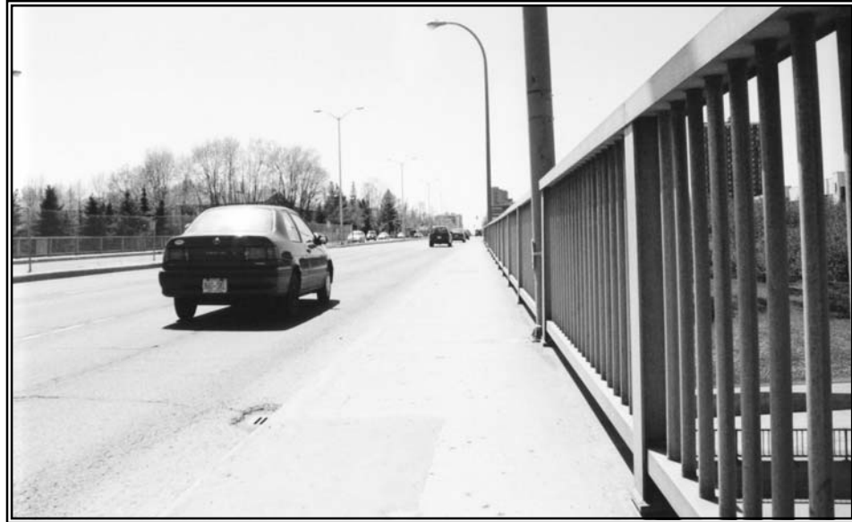
Figure 8.28 Bridge over Ottawa River Parkway, Carling Avenue Photo: C. Fullerton
