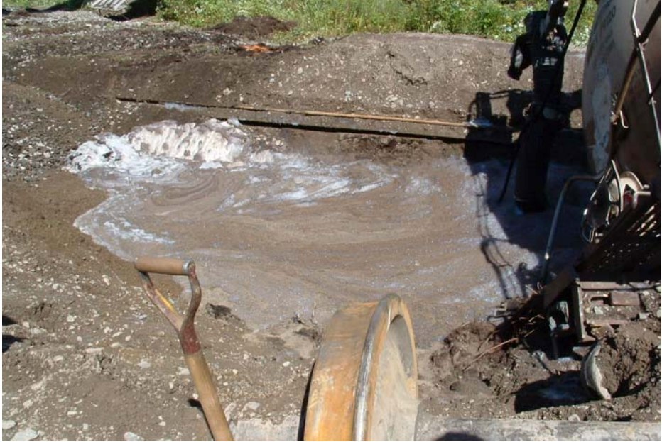
Figure 2.18 : Settlement feature which led to derailment of train at the Lévis subdivision site in 2004 (Konrad et al. 2007)
