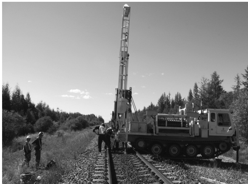
Figure 3.6 : Surface conditions at Mile 102.0 during installation of instrumentation.
