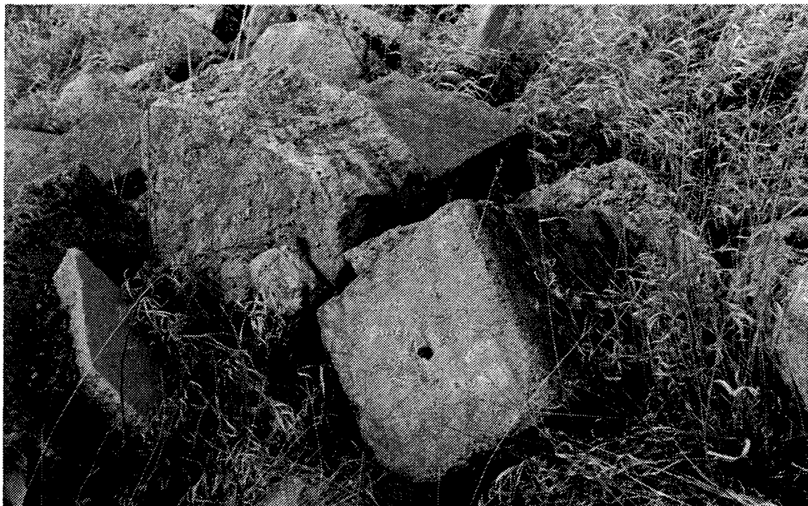
Figure 5.18 Rosthern brickyard site, concrete debris.
