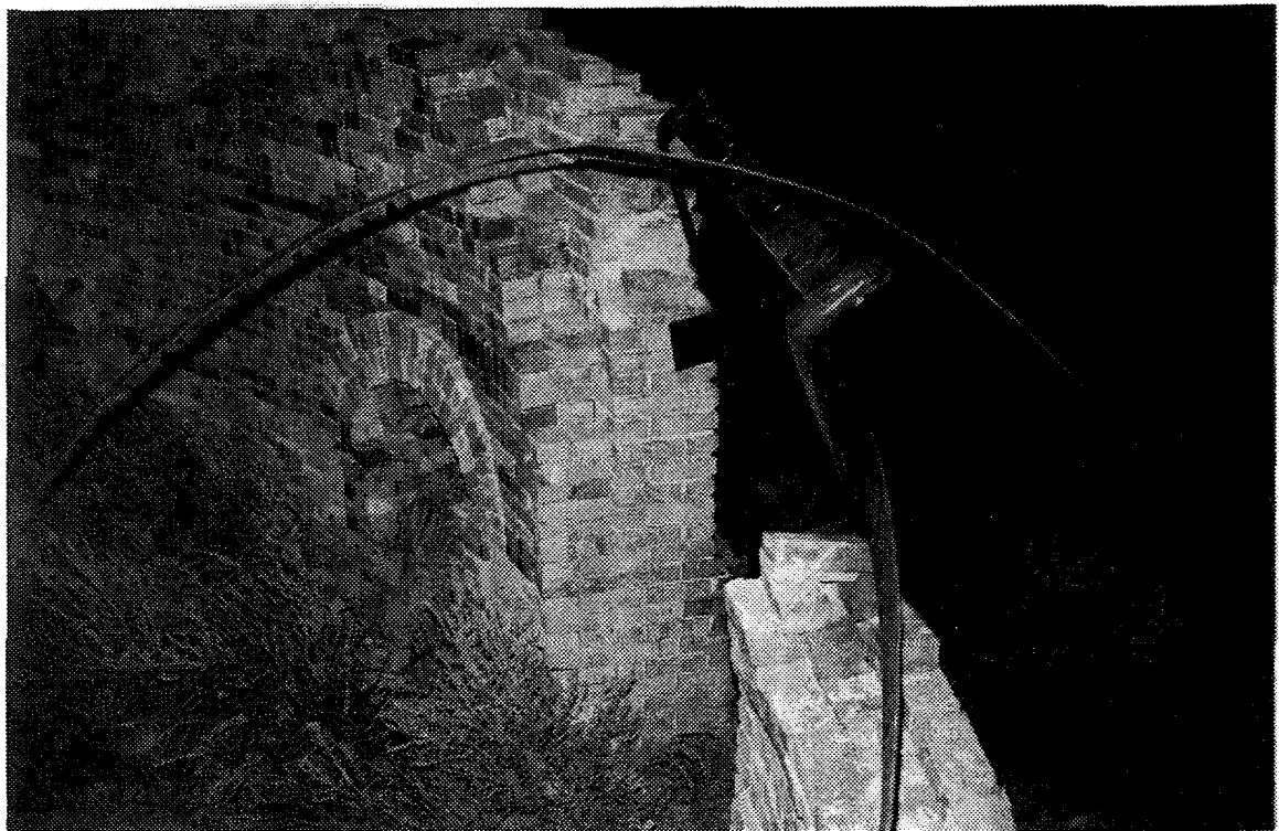
Figure 6.47 Boundary Dam site, detail of collapsed kiln in 1995.
