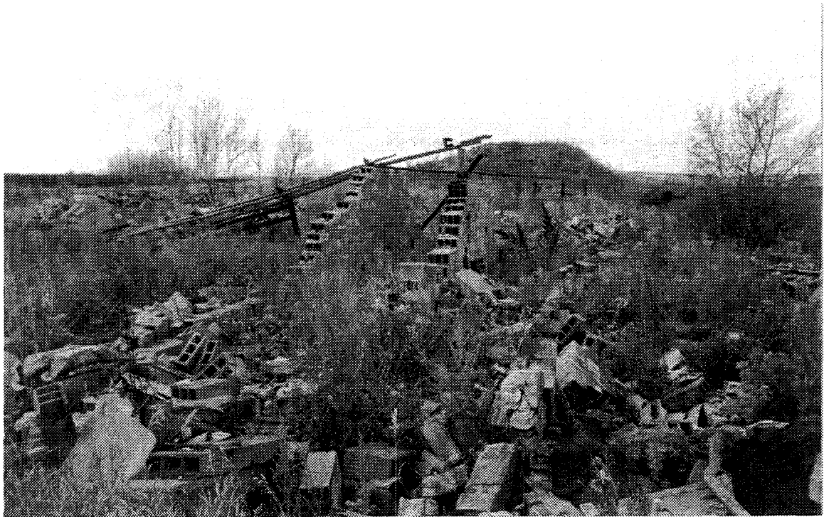
Figure 6.4 Remains of drying tunnels at the Bruno site in 1995, made from Bruno structural tile. Facing west with last clay pile in background.
