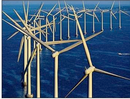
Offshore wind farm. Source: http://www.sulangaenergy.com/images/wind-turbines-370-x-283.jpg
