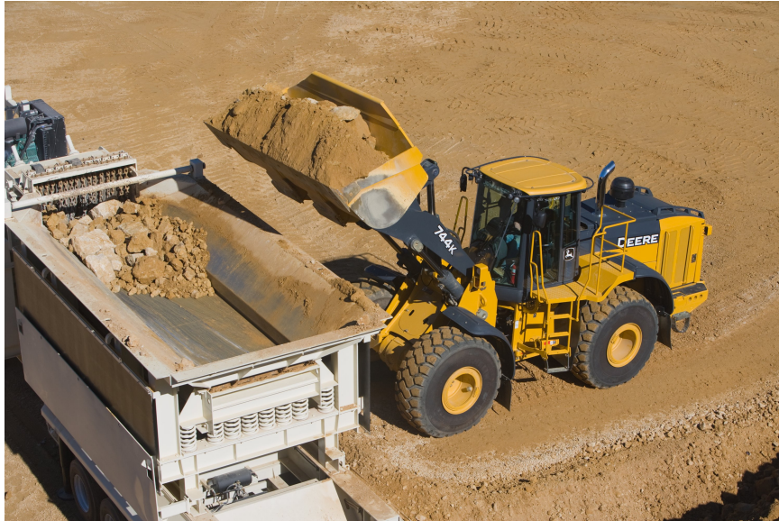
Figure 2.3: Deere 744K Loading A Crusher
