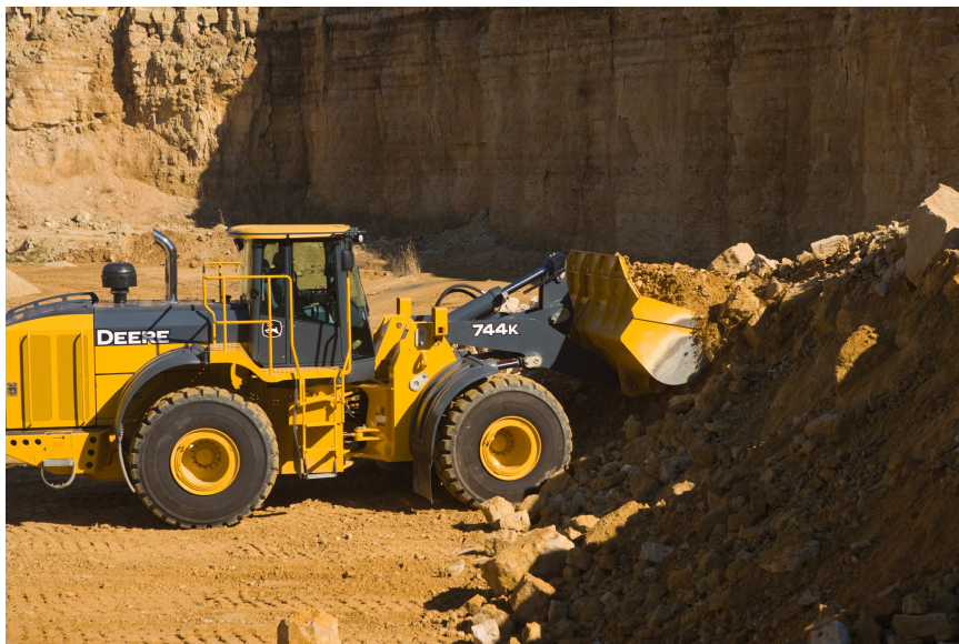
Figure 2.2: Deere 744K Face Excavating
