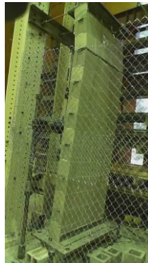
Figure 4.59: Crack position of ID3
