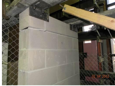
Figure 4.30: Cracking below the top course of block in Specimen RD1
