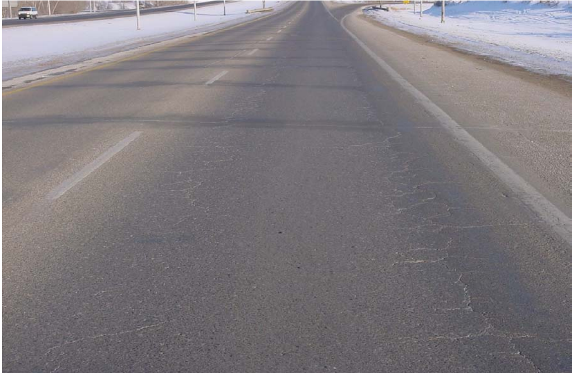
Figure 2.1 Fatigue Cracking of Asphalt Concrete
