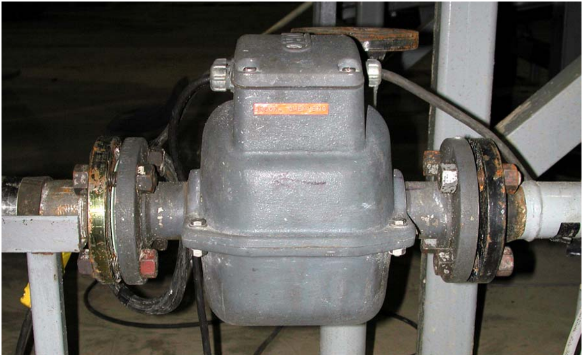
Figure F.18: 2 inch Foxboro magnetic flowmeter on the 53 mm feed pipe used in the 156.7 mm flume experiments
