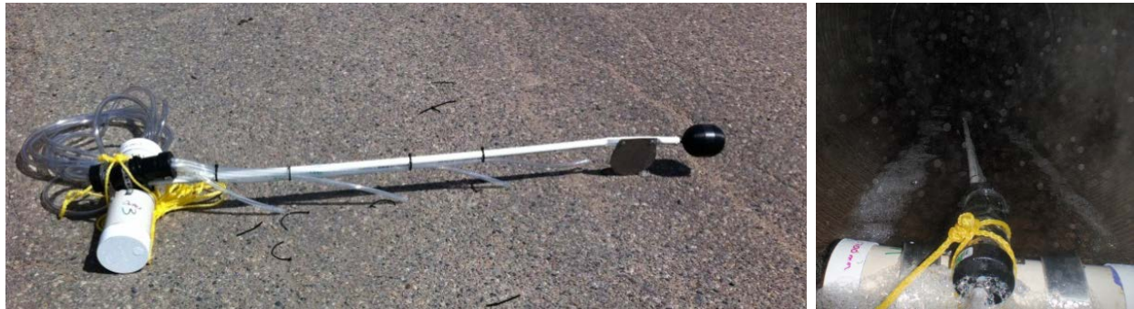
Figure 3-5. Adapted intake strainer design (left) initially used for project shown in the inlet pipe at the bottom of the manhole (right).
