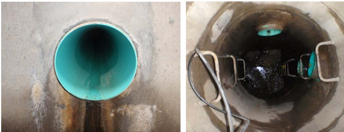
Figure 3-7. Pipe (left) conveys stormwater from the catchment area to the manhole (right, top-down view).
