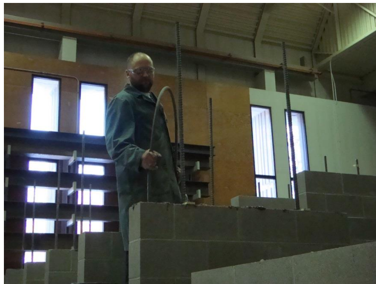
Figure 3.14. Pencil vibration of grout
