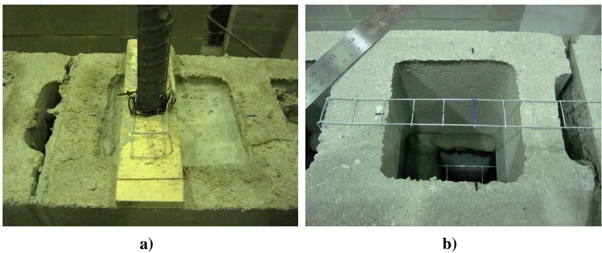
Figure 3.16. Placement of top bars: a) use of plywood and tie wires, and b) guide wire used to place No. 20 reinforcing bars in specimens
