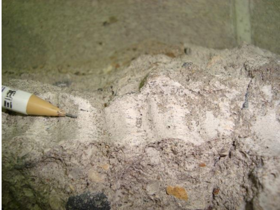
Figure 4.13. Scraping of reinforcement lugs on surrounding grout in splice region, specimen W800(No.25)-3.5-3
