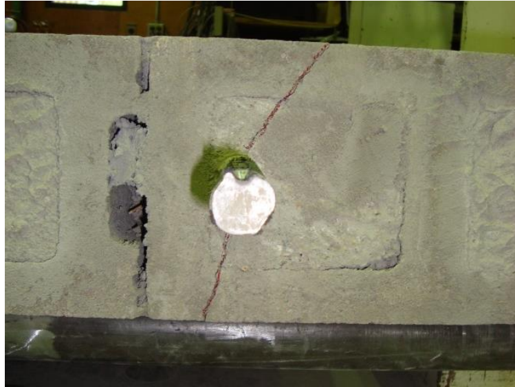
Figure 4.10. Splitting of grout surrounding reinforcement on W800(No. 25)-3
