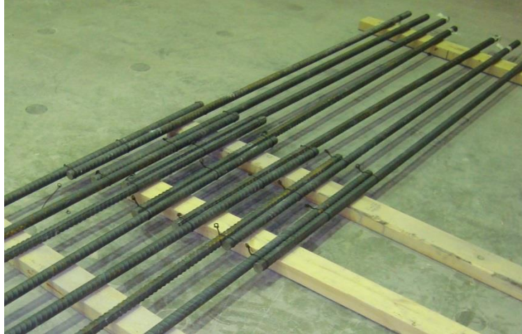
Figure 3.18. Lap spliced reinforcement connected using tie wire
