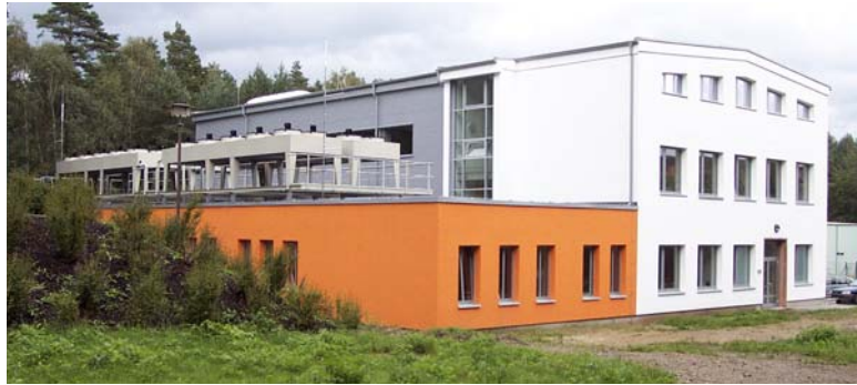
Fig. 3: TOPFLOW building with dry cooling system on top of the roof of the left wing
