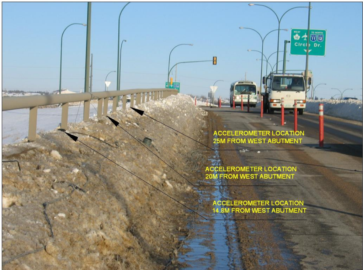
Figure 3.6. Closed lane during testing.
