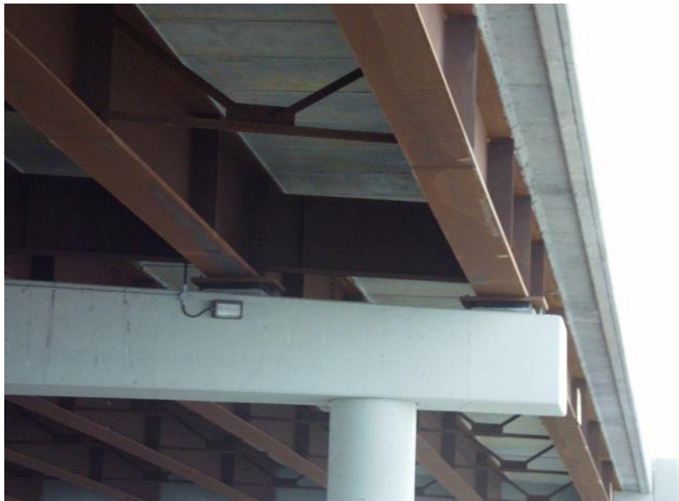
Figure 3.5. Connection between girders and pier.
