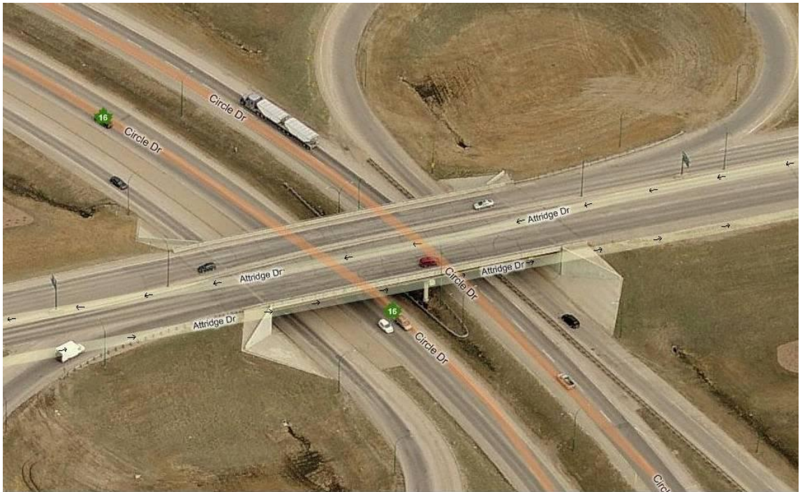
Figure 3.1. Aerial view of the Attridge Drive Overpass (Source: Microsoft Bing Maps).
