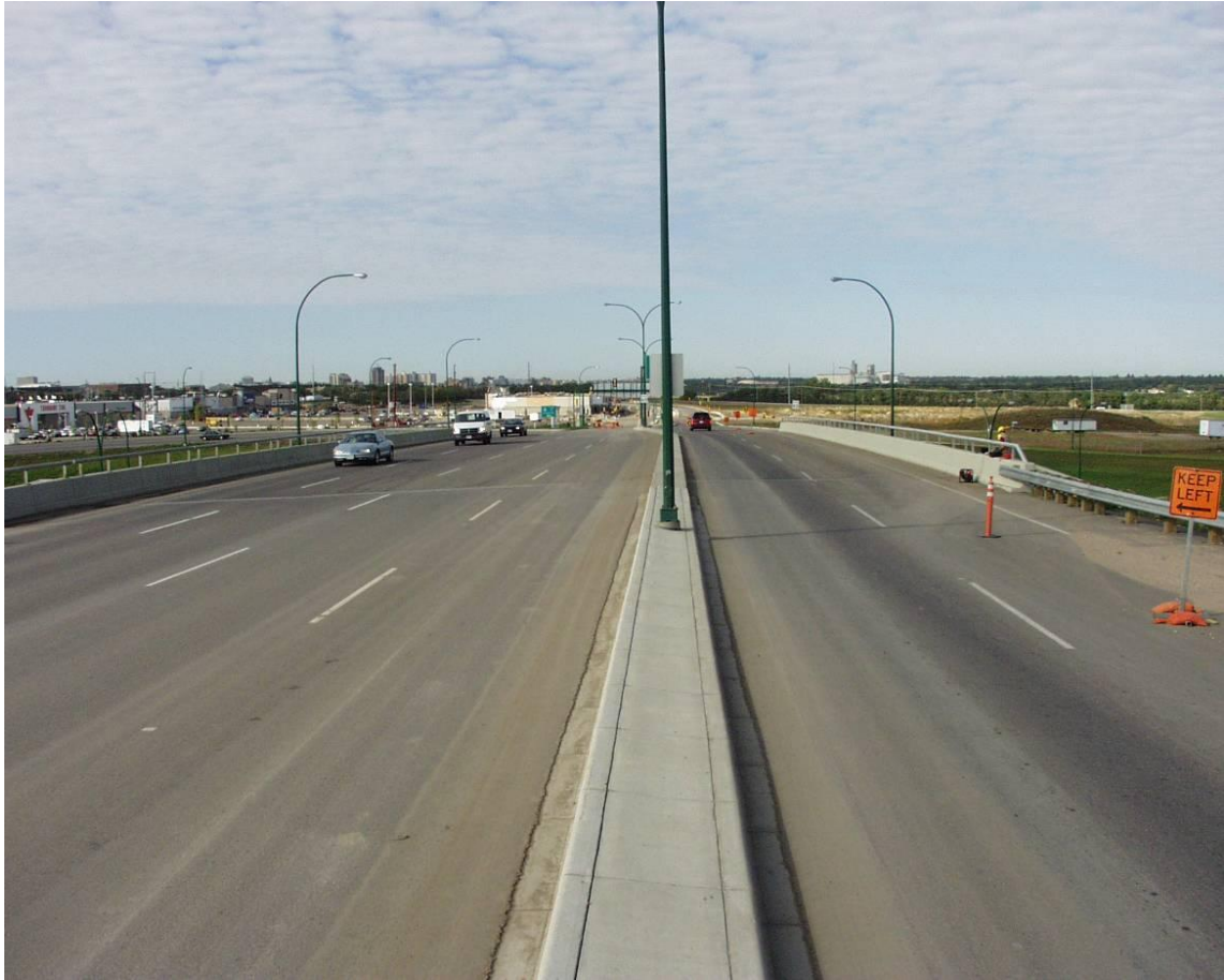
Figure 3.3. Driving lanes, viewed from the East.
