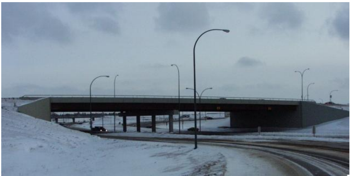
Figure 3.2. Attridge Drive Overpass, viewed from the north side.
