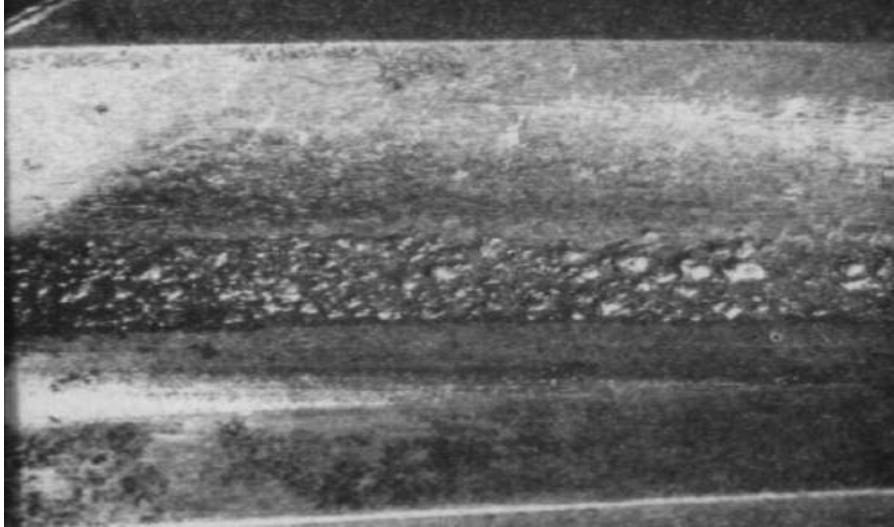
Figure 1-1 Fatigue failure of the tooth surface
