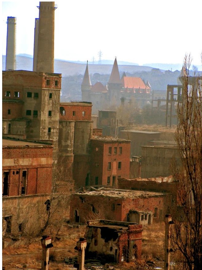
Figure 6.1 View of the former Hunedoara Steel Plant. (Photo 2008).
