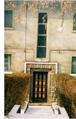
Figure 4.8 Collective dwellings, Hunedoara (1949-1951), Entrance detail. Architects D. Hardt et al. (Photo 2008).
