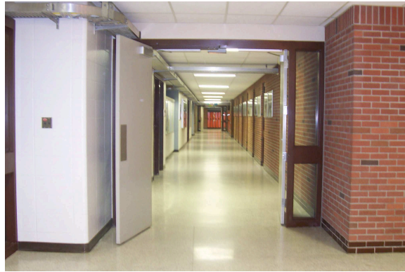
Figure 4.4: One of the hallways where the testing was done
