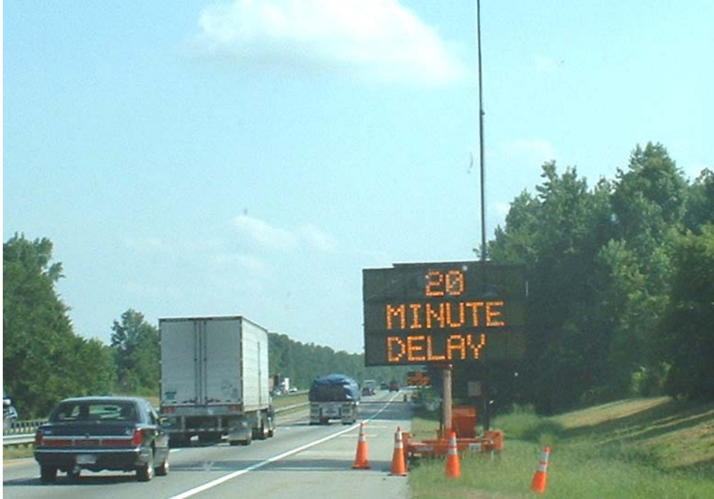
Figure 5: Road Side Message Sign Advising Motorists of Delay Ahead
