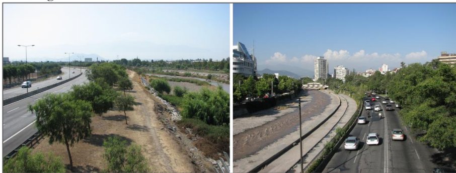
Figure 6.13: Costanera Norte (left) and Andres Bello Avenue (right) flanking the riversides.
