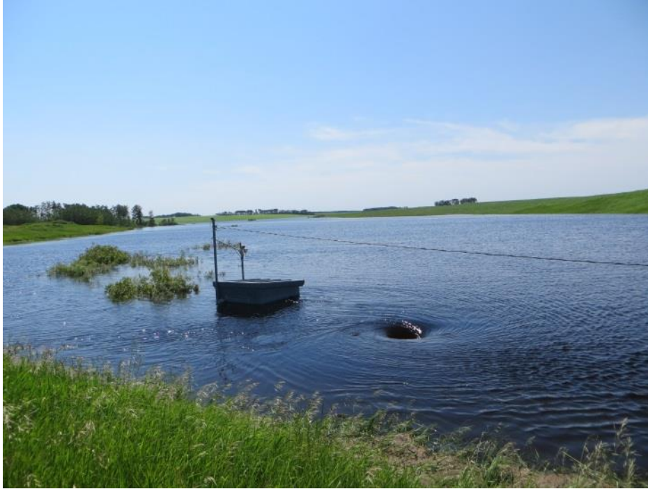
Figure B.7: Outlet of SCRБ looking upstream on July 4, 2014 approximately 3 days after record breaking peak flow occurred from rainfall. Photo credit: Stacey Dumanski.
