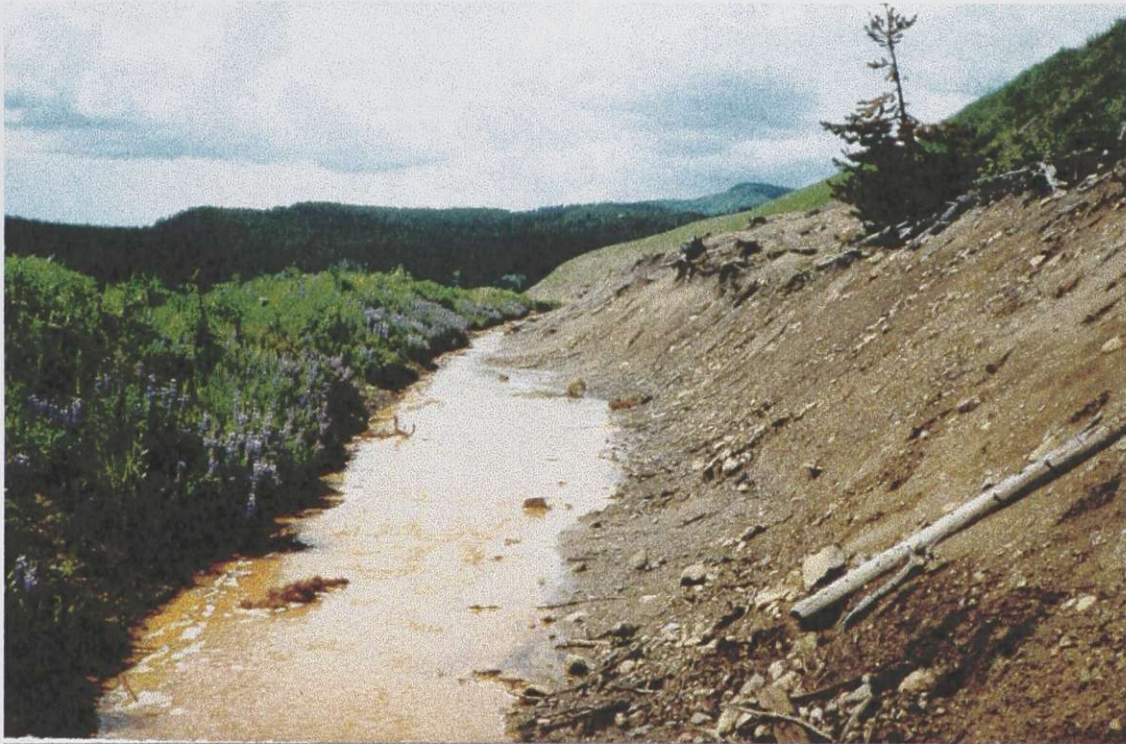
Figure 1.7 Acid rock drainage collection ditch.
