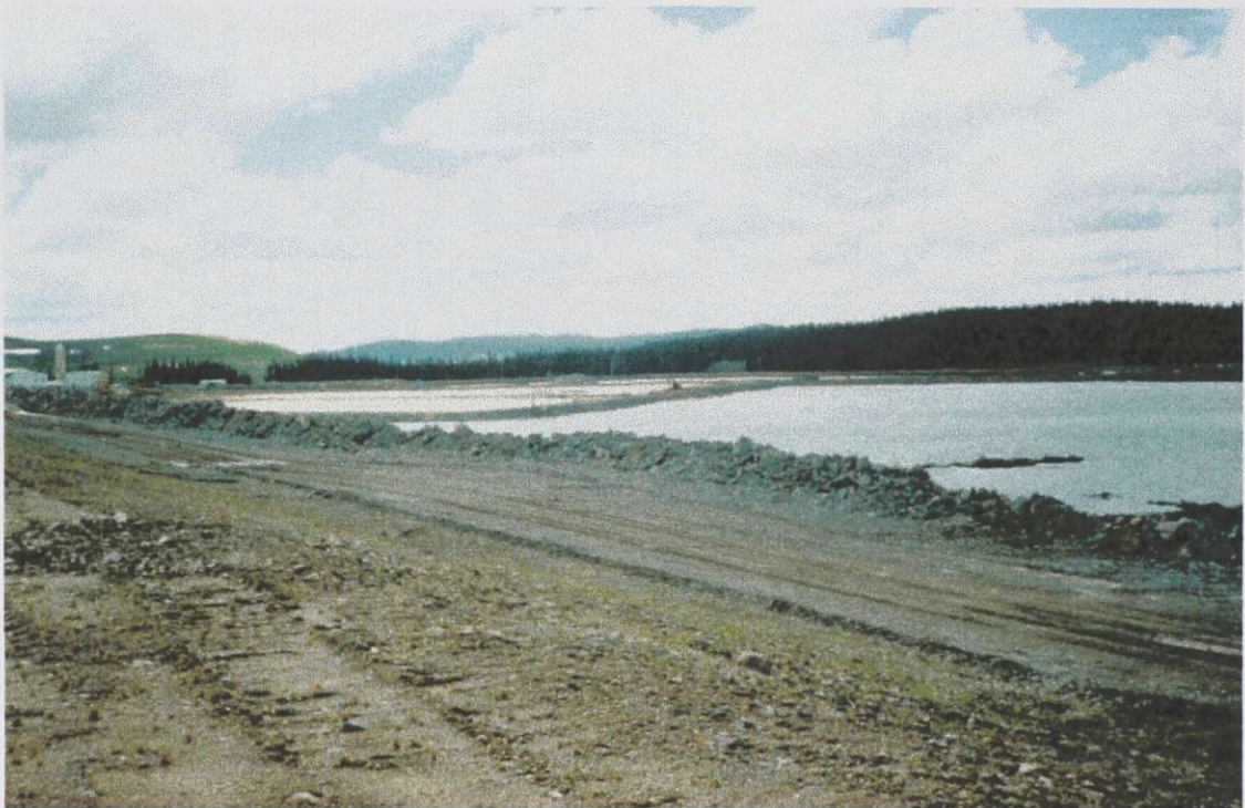
Figure 1.3 Diversion and Sludge Ponds and the Water Treatment Plant.
