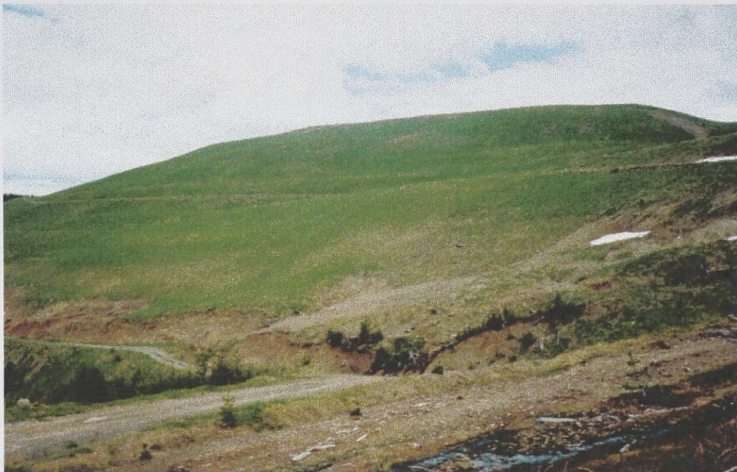
Figure 1.6 Main Dump after till cover placement.
