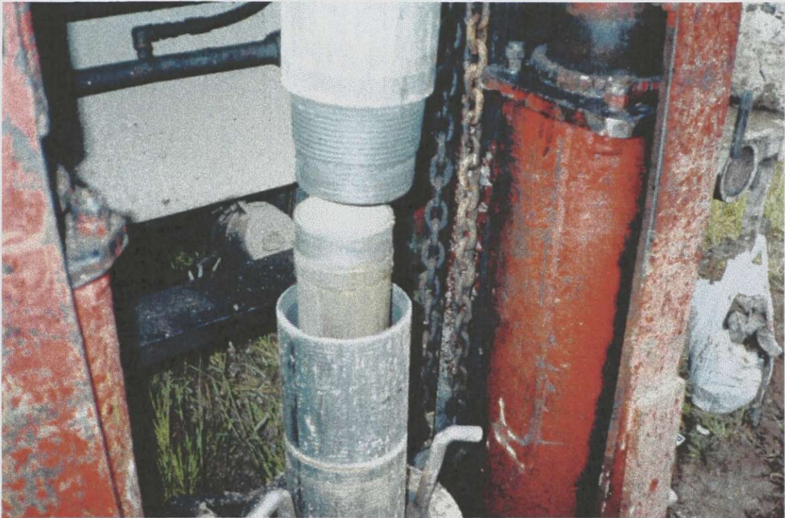
Figure 4.2 Doubled walled casing construction.
