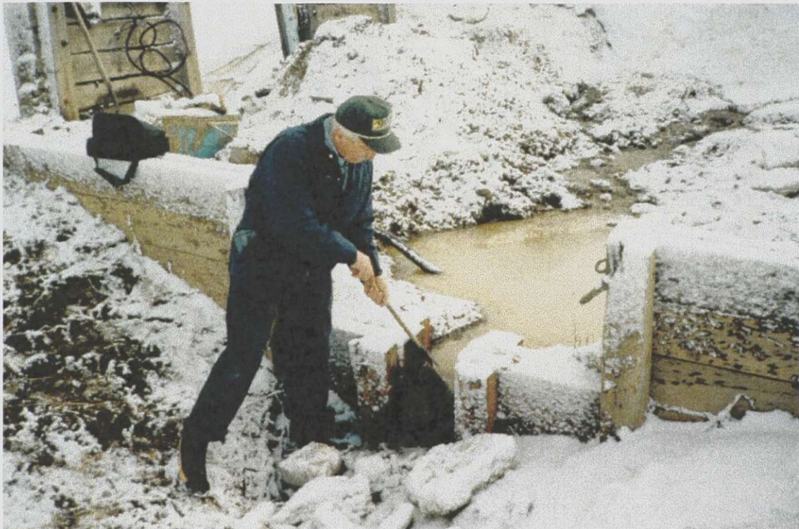
Figure 4.12 Weir flow instrumentation (R 98-03 station).
