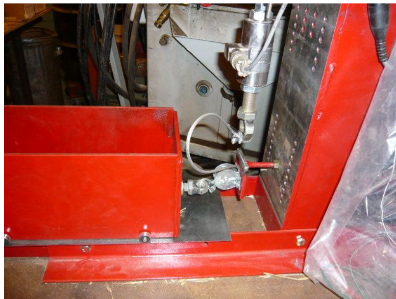
Figure B.6 Photograph showing the position of the box and cable when the “zero” value is accepted in the Labview program.
