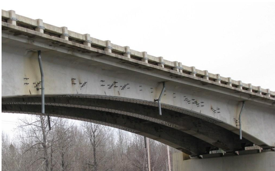
Figure 3.18 Steel plate strengthening of Hudson Bay bridge after completion.
