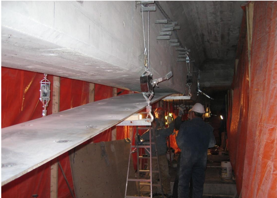
Figure 3.17 Steel plate strengthening of Hudson Bay bridge during installation.
