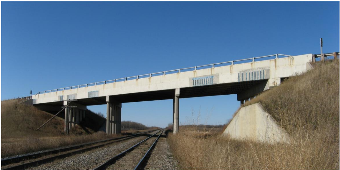
Figure 3.21 Photograph showing the Broadview bridge (looking north).
