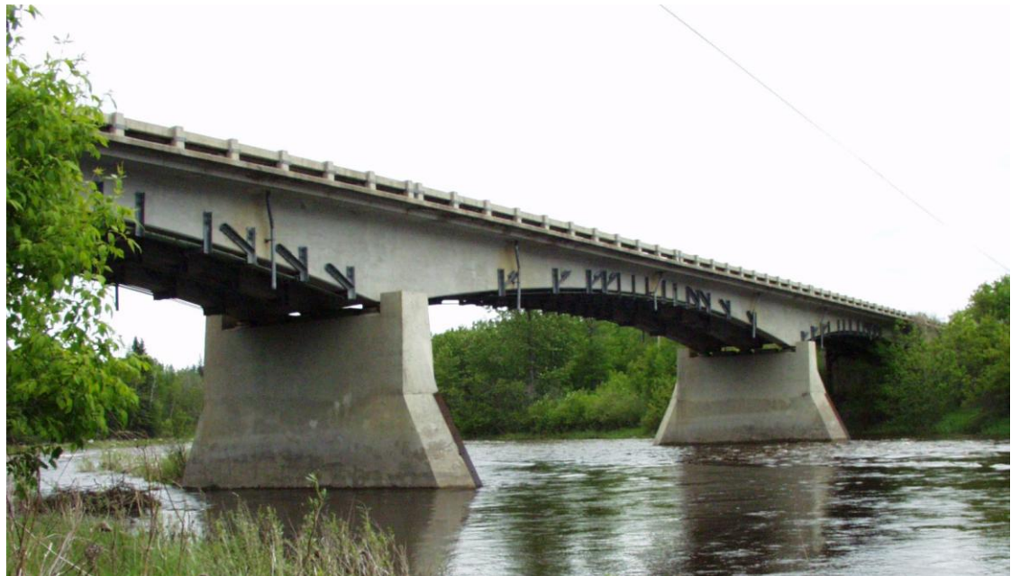
Figure 3.2 Bridge photograph showing external positive moment reinforcement.
