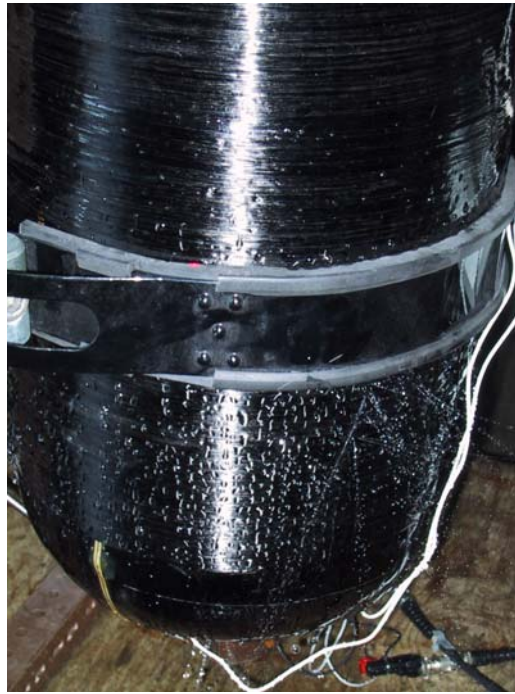
Figure 6.2: Tank Fatigue Failure
