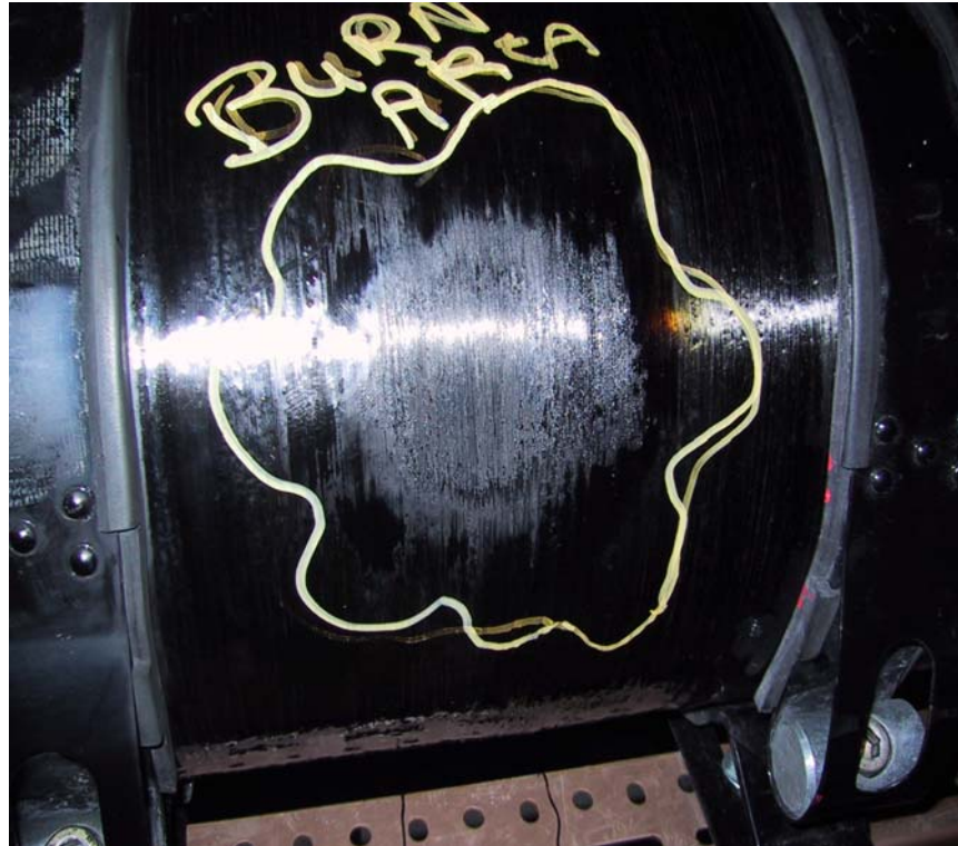
Figure 6.9: Heat Damage on Tank Sidewall
