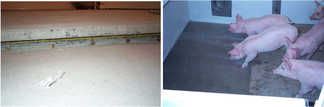
a) Nozzles for the washing gutter b) Operation of the nozzles
