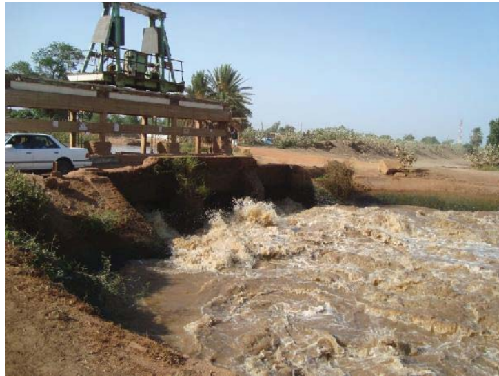
Figure 2-11. The Basatna regulator hydraulic structure 99 km from the Sennar Dam
