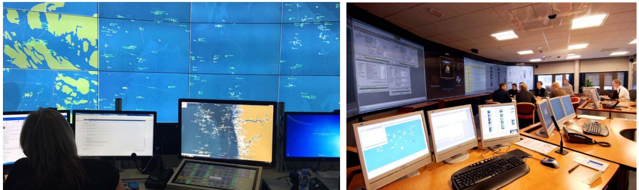
Figure 109. The logistics and emergency operations center (Source: Equinor.com)
