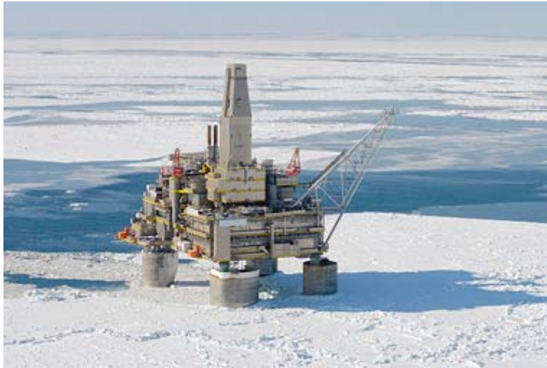
Figure 88. Piltun-Astokhskoye-B oil production platform (Source: Sakhalin Energy).
