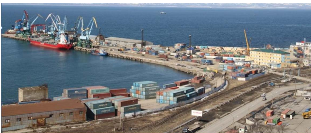
Figure 82. The Korsakov shore base on Sakhalin (Source: Sakhalin-Shelf-Service, LLC).
