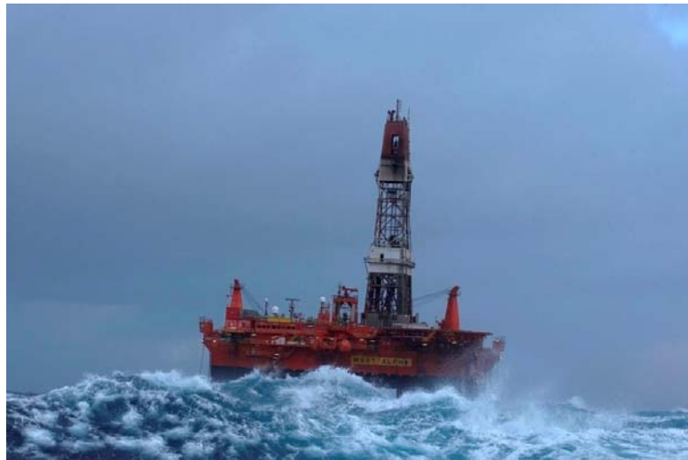
Figure 60. The West Alfa drilling rig in the Kara Sea (Source: Livejournal.com)
