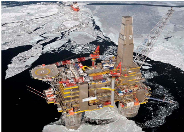
Figure 89. Lunskeye-A gas production platform (Source: Sakhalin Energy).
