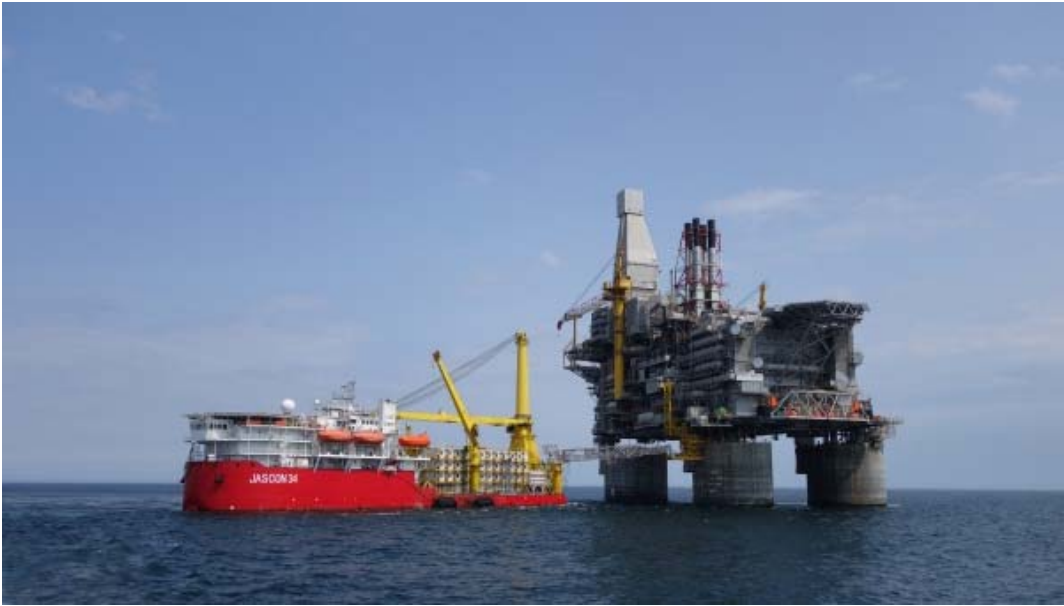
Figure 74. Jascon 34 vessel near “Berkut” platform (Source: offshoreenergytoday.com)
