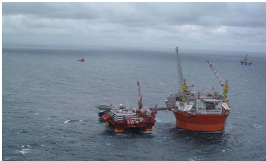
Figure 26. Goliat FPSO preparations in full swing (Source: Offshoreenergytoday.com)
