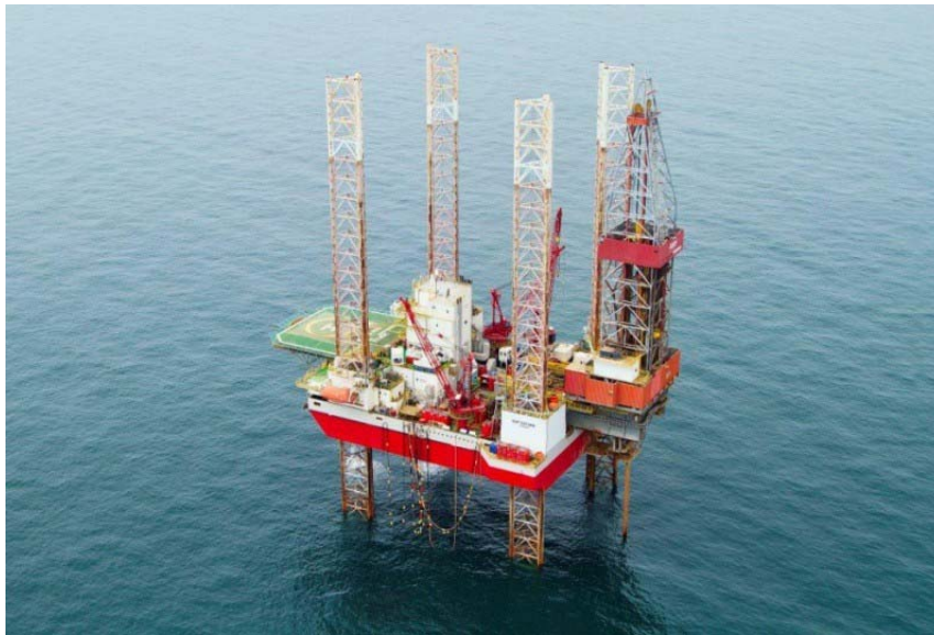
Figure 68. The GSP Saturn rig (Source: GazpromNeft-Sakhalin).
