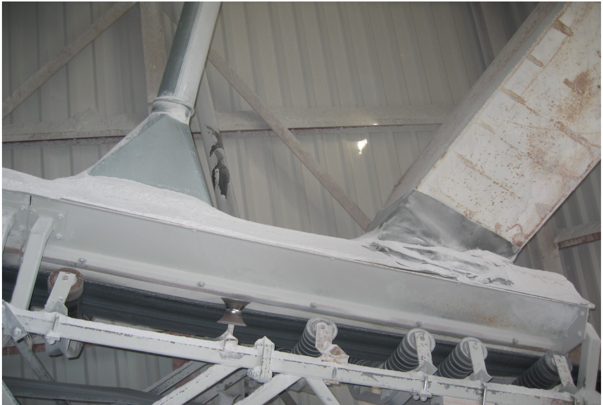
Picture 1. Example of a picture taken during an inspection
