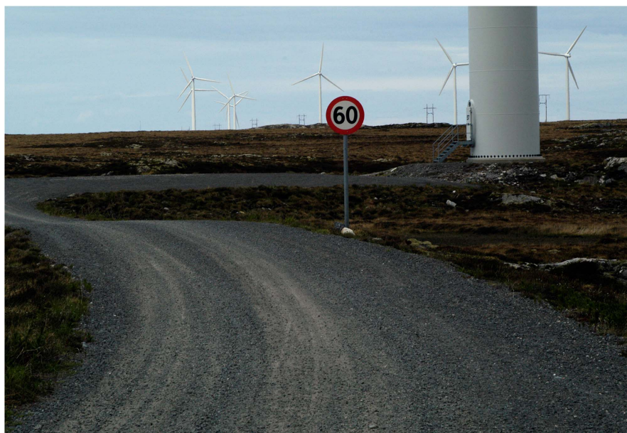
Fig 4. Access roads through the wind farm (photo by Ilan Kelman).
