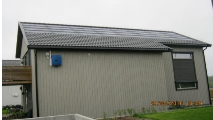
Figure 17: View of a typical house in Skarpnes, with solar PV on the rooftop
