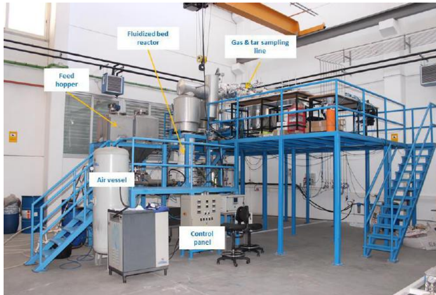
Figure 3.8: Pilot scale gasification system at University of Zaragoza, Spain
