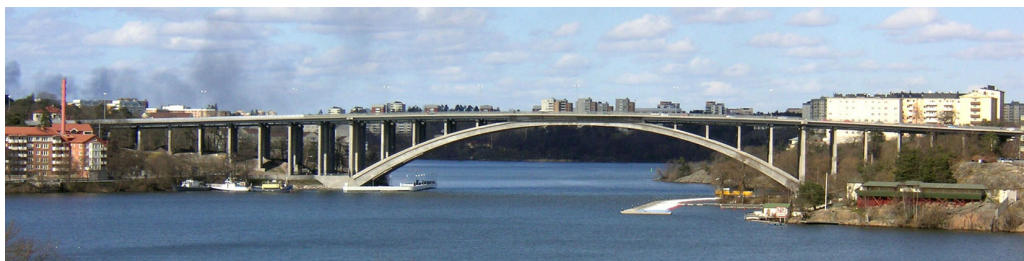
Figure 2.15: Traneberg bridge, Stockholm (1934)
