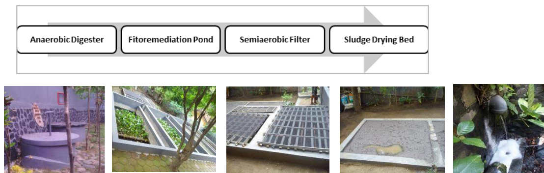
Figure 4. Condition Processing Unit WWTP Tlogomas
