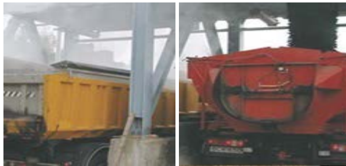
(a)HMA (b)WMA Plate 1.1 Asphalt Mixing Plants (Shell, 2011)
