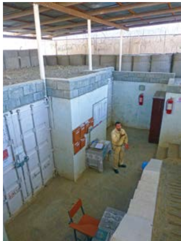
A below ground level ammunition storage facility in Bagram, Afghanistan, constructed by The HALO Trust. Image courtesy of The HALO Trust.
