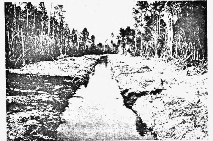
Stream "improvement" by channelization.
