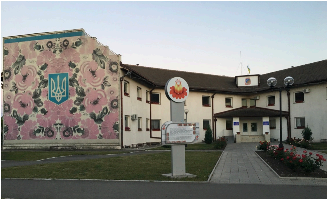
Figure 2.5 Building of the Petrykivka townhall. Photo by Iryna Voloshyna.
