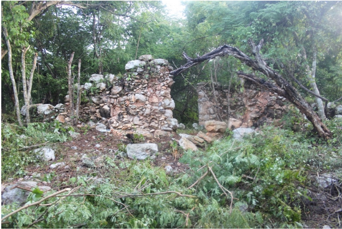
Figure 8.1 Remaining Masonry Walls of the Rancho Kiuic's Schoolhouse, Thought to be the Site of Catherwood's "Casa Real"
