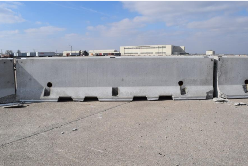
Figure 78. Barrier No. 6 Damage, Test No. NELON-1
