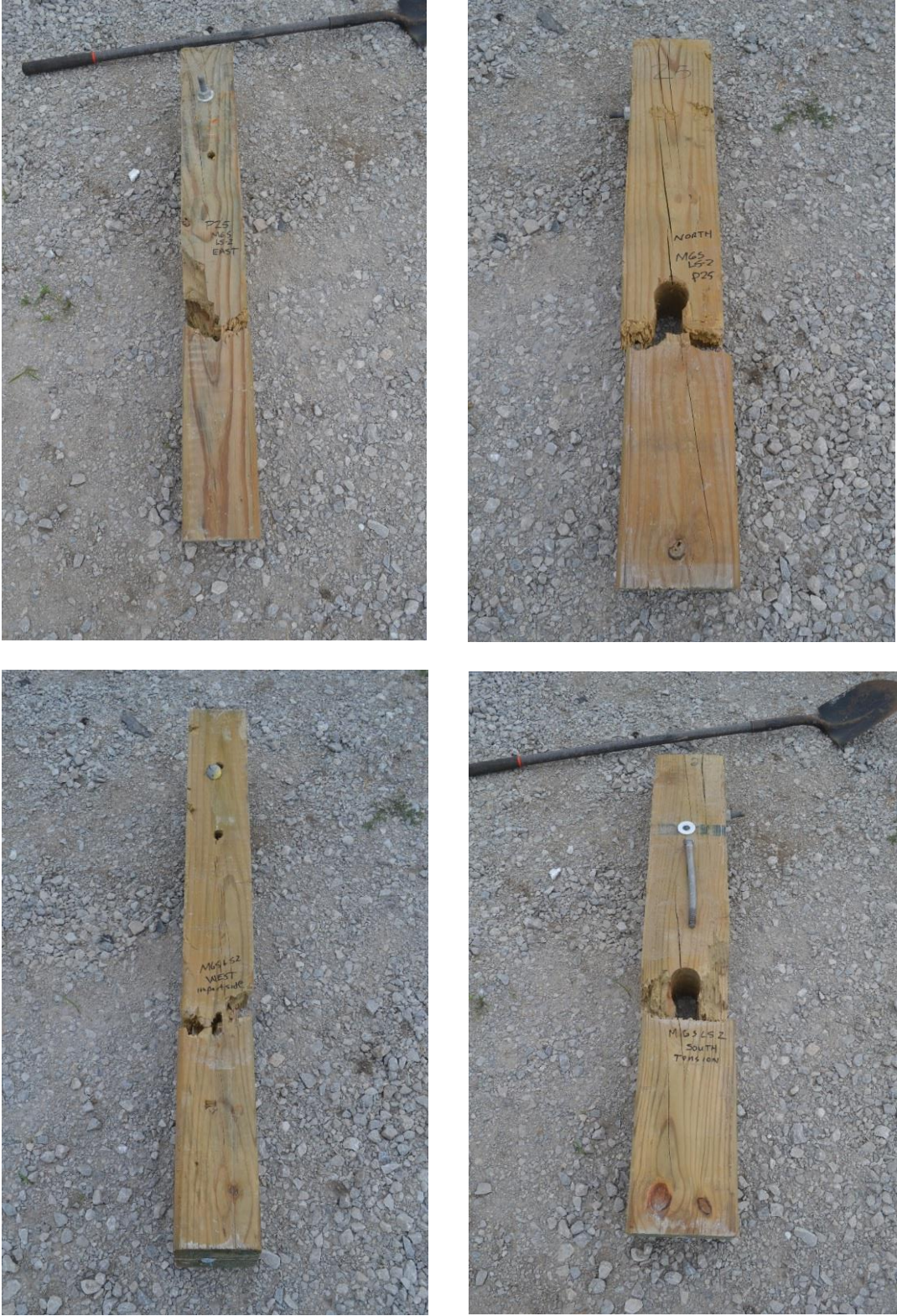
Figure 9. Post No. 25 Damage, Test No. MGSL-2
