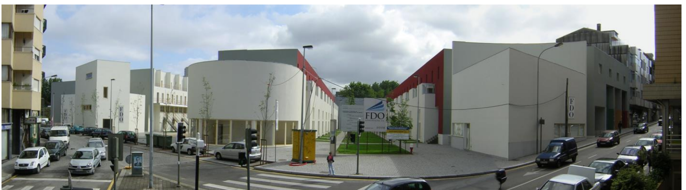
Image 4 – Bouça SAAL housing, after the 2006 renewal operation (E. F., 2006).
