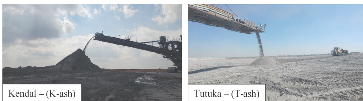
FIGURE 3.1. Fly ash being disposed of at Kendal and Tutuka power stations
