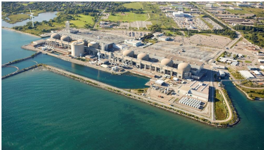
Figure 3. Pickering Nuclear Power plant (from SNL-Lavalin Website)
