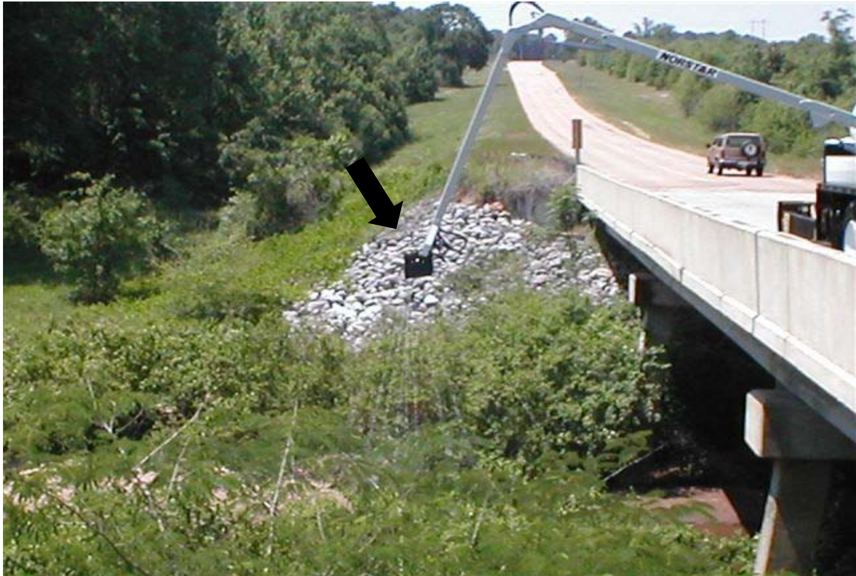
Figure 2. Long Shot boom with “nutating” head used to treat brush under bridges.
