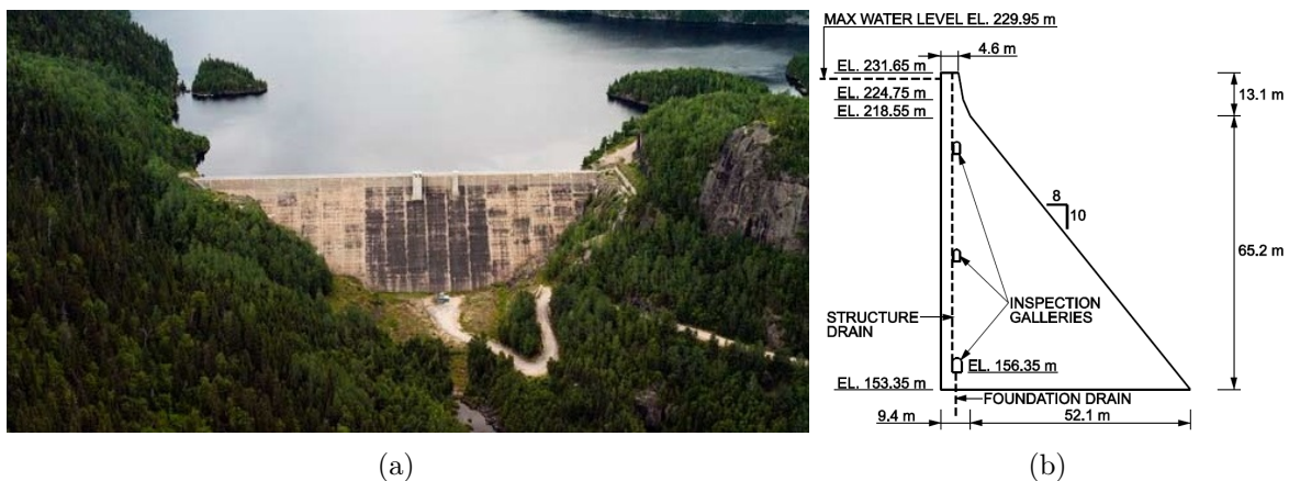
Figure 1.2 Case study dam: (a) aerial view of the dam [1] and (b) cross section
