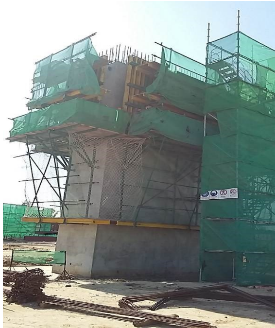
Fig.5.11 – Pier S9 with the formwork stripped
