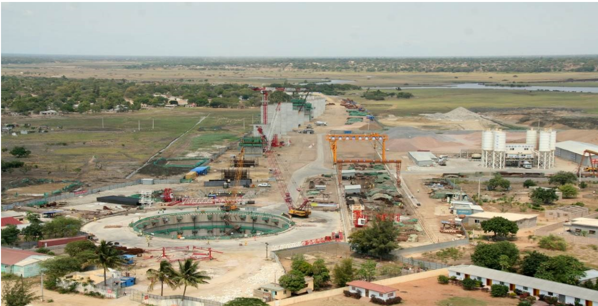
Fig.3.7 – South Bank Anchorage under construction
