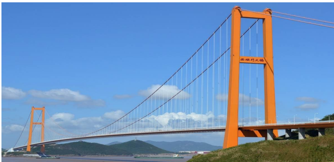
Fig. 2.2 - Xihoumen Bridge, China [2]
