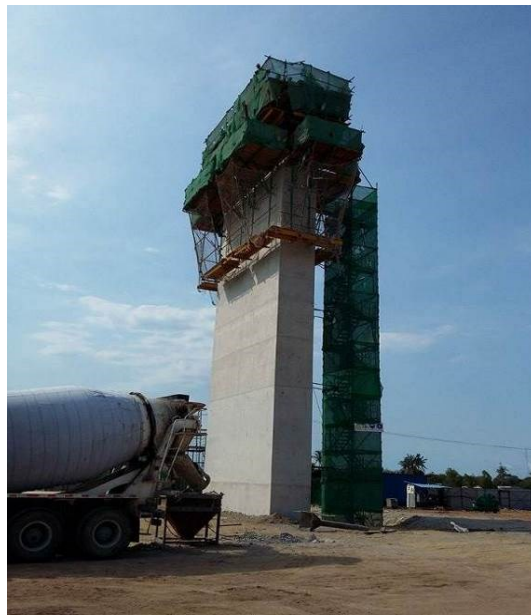
Fig.5.9 – Pier S18 with the preparation for casting
