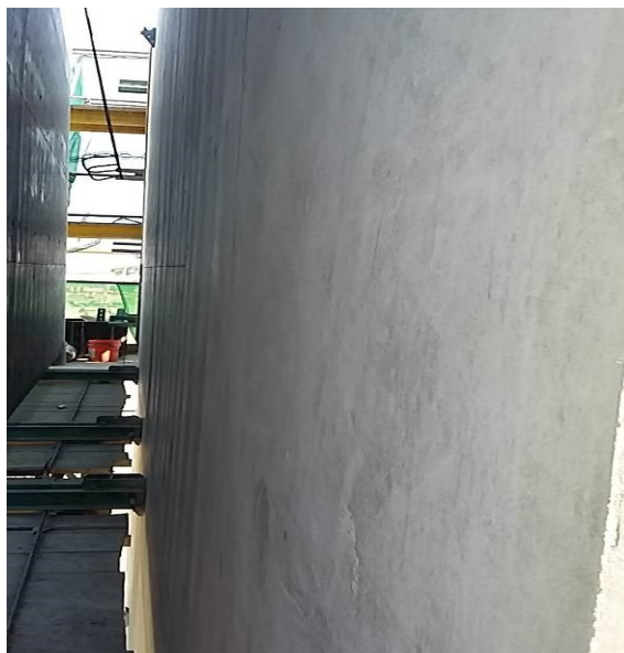
Fig.5.12 – Pier S9 with the repair works finished
