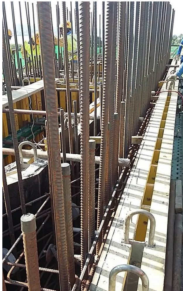
Fig.5.7 – Pier S10 with the formwork installed and ready for concrete casting
