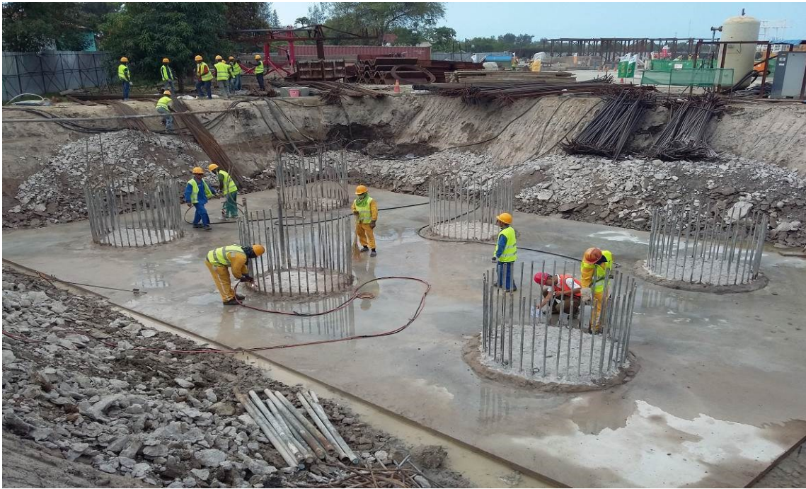
Fig.3.11 – Pile Head regularization for installation of Pile Cap Reinforcement – Pier S5
