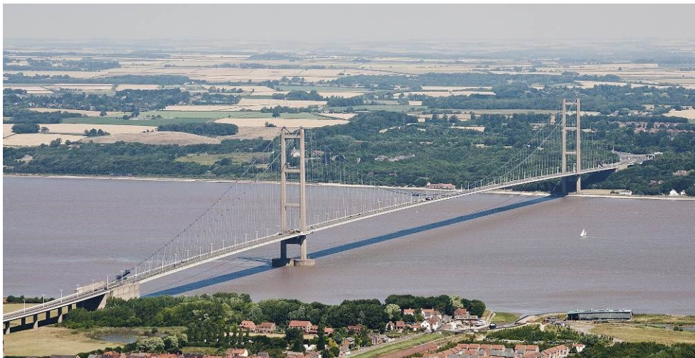
Fig. 2.8 – The Humber Bridge, England, UK [8]
