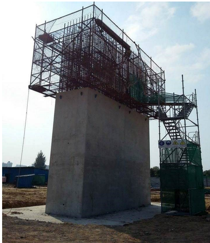
Fig.5.4 – Pier S8 with the operation platform settled
