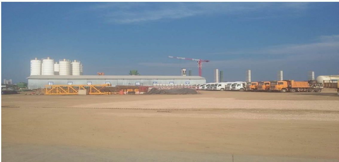
Fig.4.5 – Vehicle and machinery parking area (Part of the South Construction Site)
