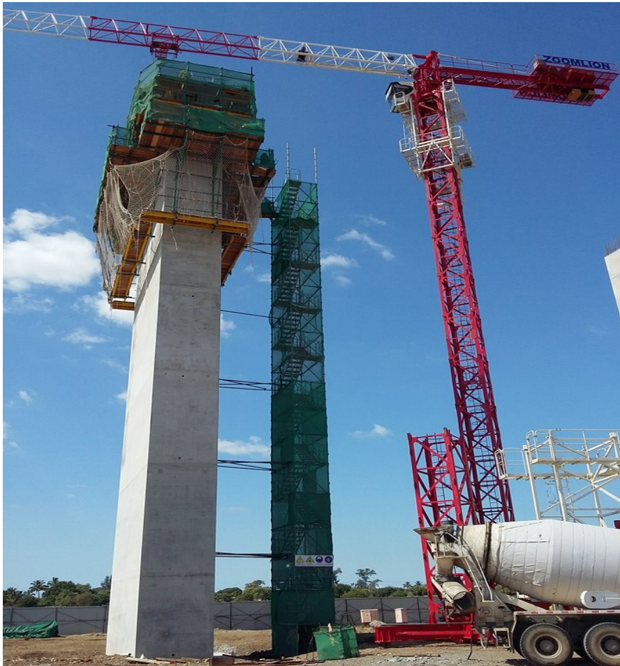
Fig.5.3 – Pier S12 with the rolling ladder and the tower crane installed
