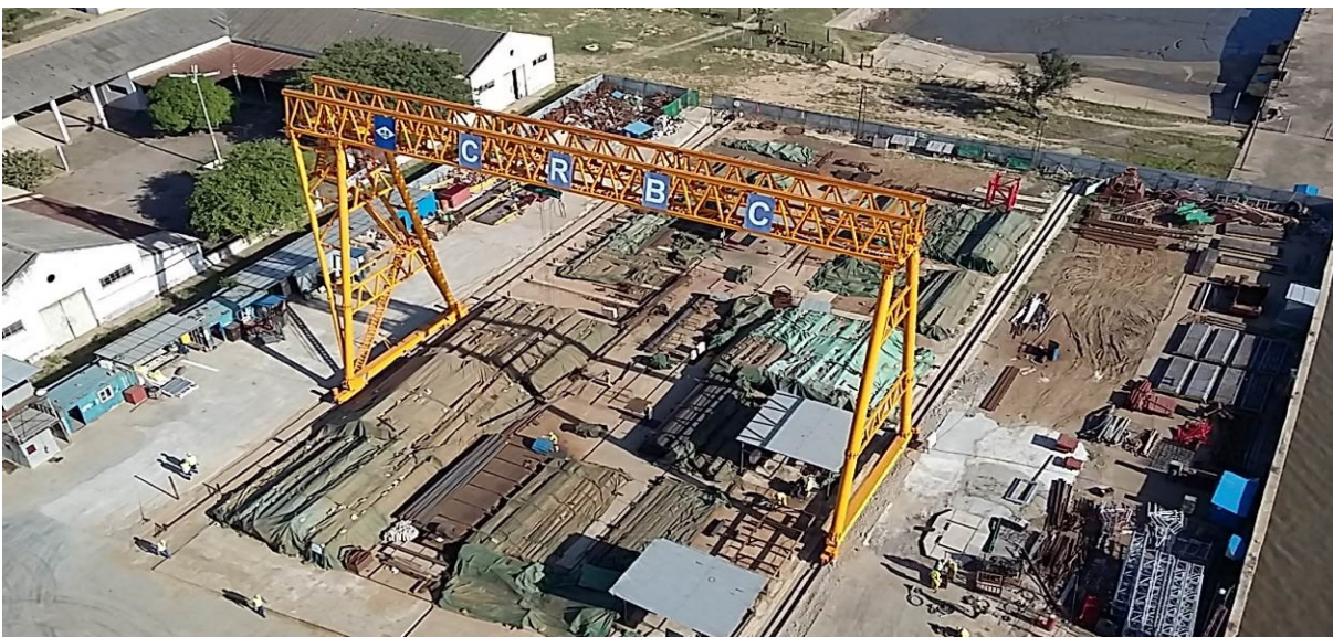
Fig.4.4 – View from Pylon M2 with the Pylon Working Area
