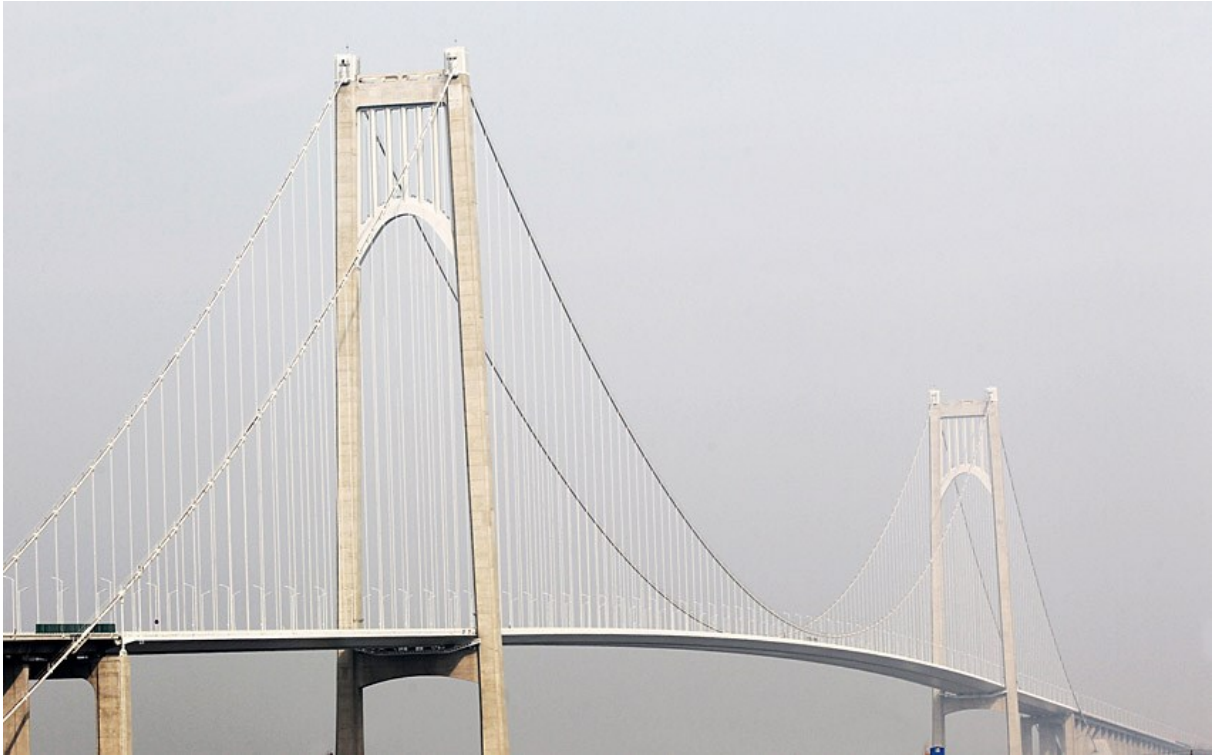
Fig. 2.4 - Fourth Nanjing Yangtze Bridge, China [4]
