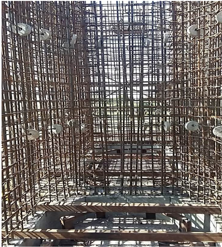
Fig.5.5 – Pier S8 with the reinforcement installed
