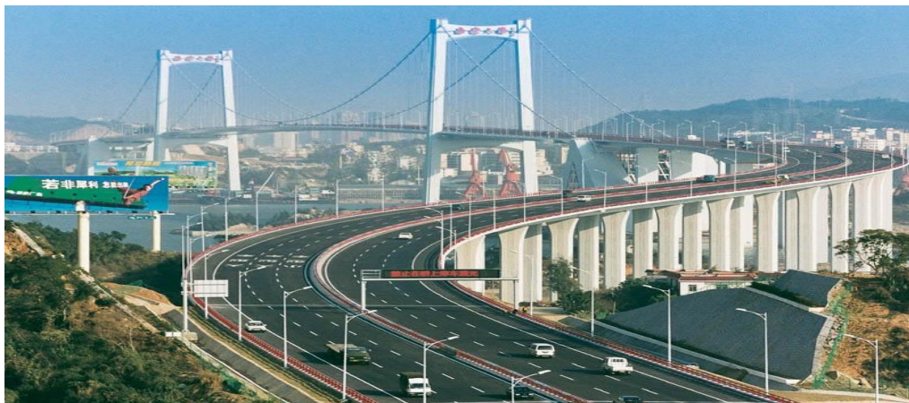
Fig. 2.6 - Xiamen Haicang Bridge (CRBC work), China [6]
