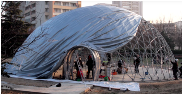
Figure 71 – Temporary Cathedral of Créteil (Paris, France), based on a gridshell composite structure (ThinkShell 2014)
