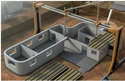
Figure 17 - Automated building construction using CC technology (Corporation, Contour Crafting 2017)
