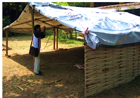
Figure 5 - Bamboo construction shelter demonstrated in Myanmar Training Course (Shelter, ReciproBoo. 2017)
