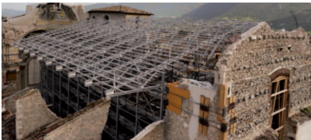
Figure 72 - Temporary Church Roof after in Italy (Mafeld and JEC 2017)
