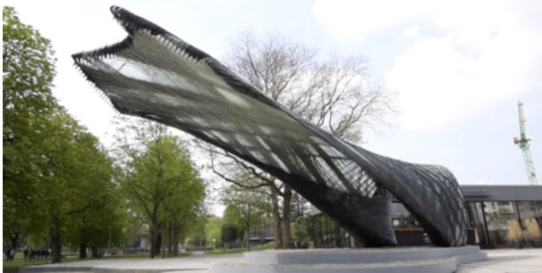
Figure 69 - A glass and carbon fibre-reinforced composites pavillion made by robots and drone. (JEC_Group 2017)
