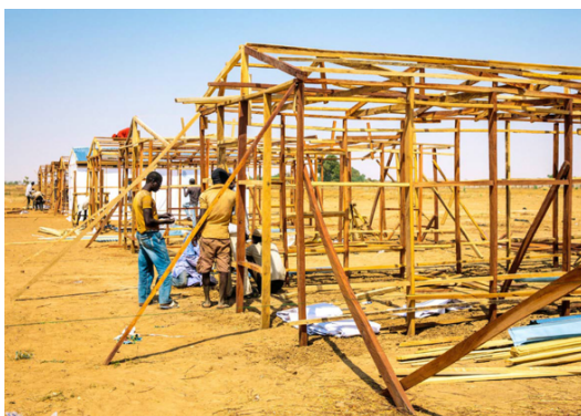
Figure 4 - Shelter construction wood structure in Maiduguri, Nigeria (© M. Mohammed, IOM 2016)
