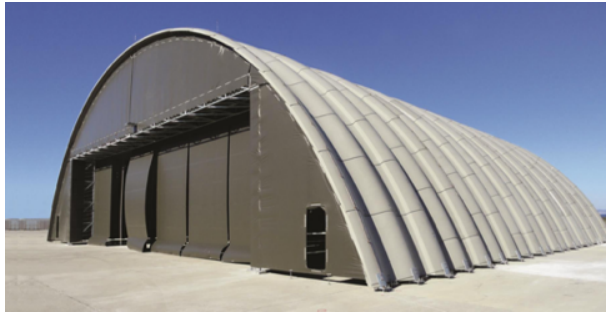
Figure 66 - Composite Modular Hangar (CMTH®) (Dasyc 2015)
