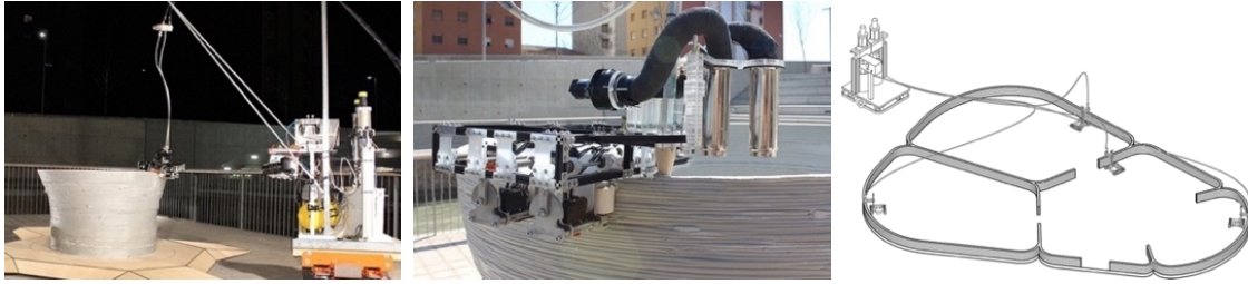
Figure 20 - Minibuilders, small robots printing big structures (IAAC 2015)
