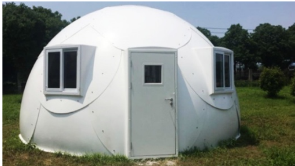
Figure 80 - Enviropod Dome Home (Enviropod 2019)
