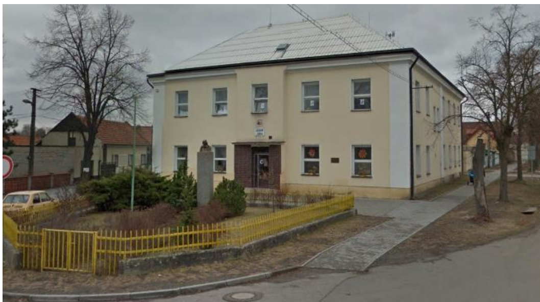
Figure 28 – Primary School (Google Street View)
